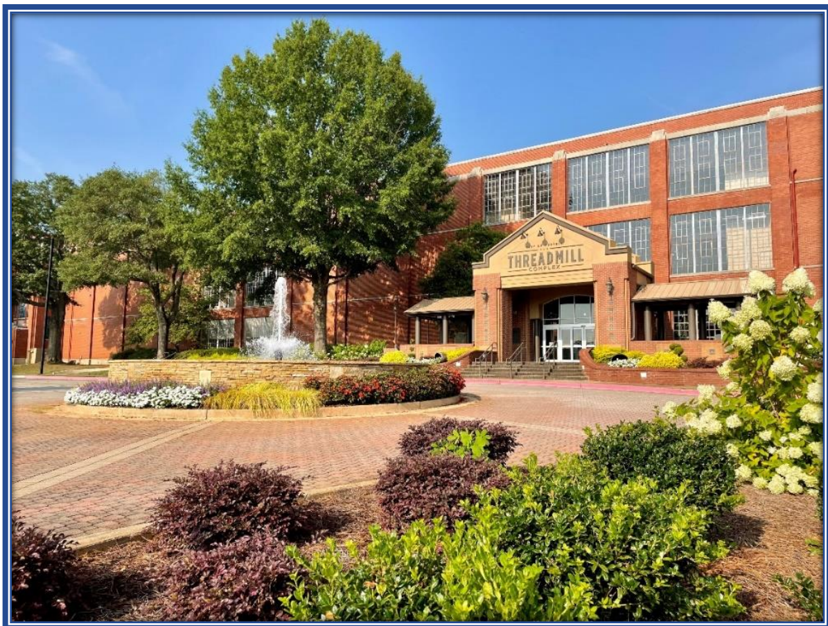
Outside View of Threadmill Complex
