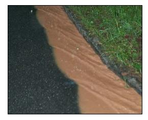
Figure 1.2 Sediment is the Most Common Stormwater Pollutant
