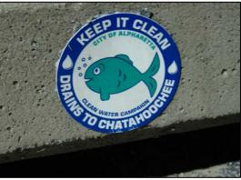
Figure 2-3 Example of a Stormwater Drain Stencil and Curb Marker
